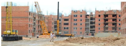
Figure 1. Construction of new 7-story houses in Sergeli district
